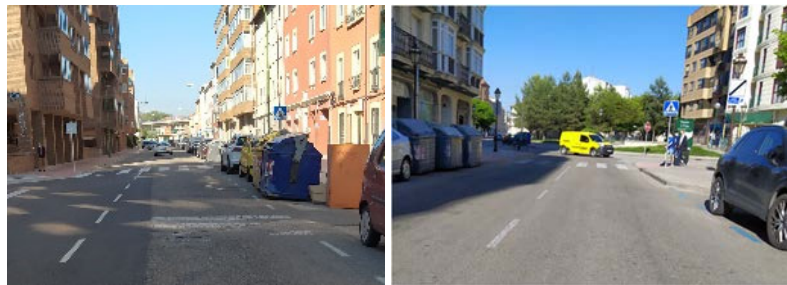
Figure 2: Examples of crosswalks with limited visibility by car parking (left) and improved by sidewalk widening (right).
