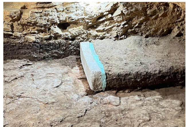
Fig. 10 Just prior to removal, expanding foam was injected into the kerf between the block and the bench and allowed to set overnight
