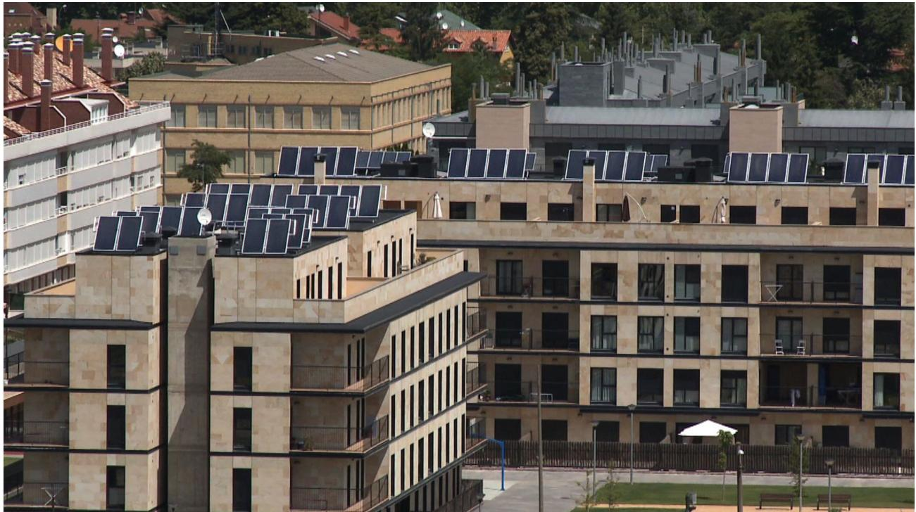
The practical use of low temperature solar thermal systems in buildings consists in using the solar radiation for heating a fluid, usually at temperatures up to 90°C.
