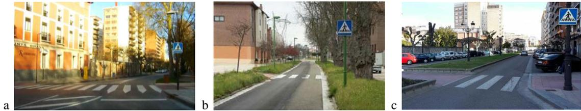
Fig. 1. (a) Raised Crosswalk; (b) Lane narrowing at P13; (c) Lane narrowing at P15.
