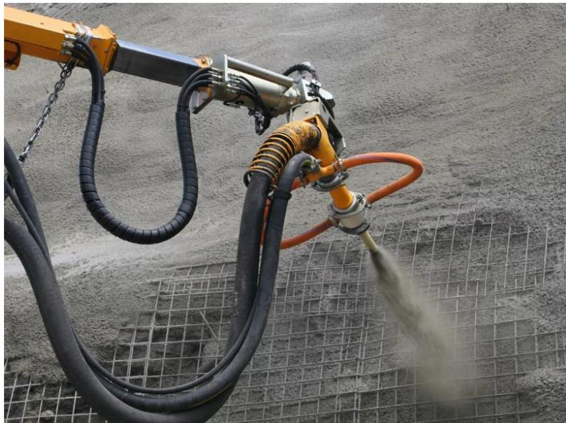
**Figure 2.1-9. Execution of lining, in this case of a slope, with projected fiber concrete.**
