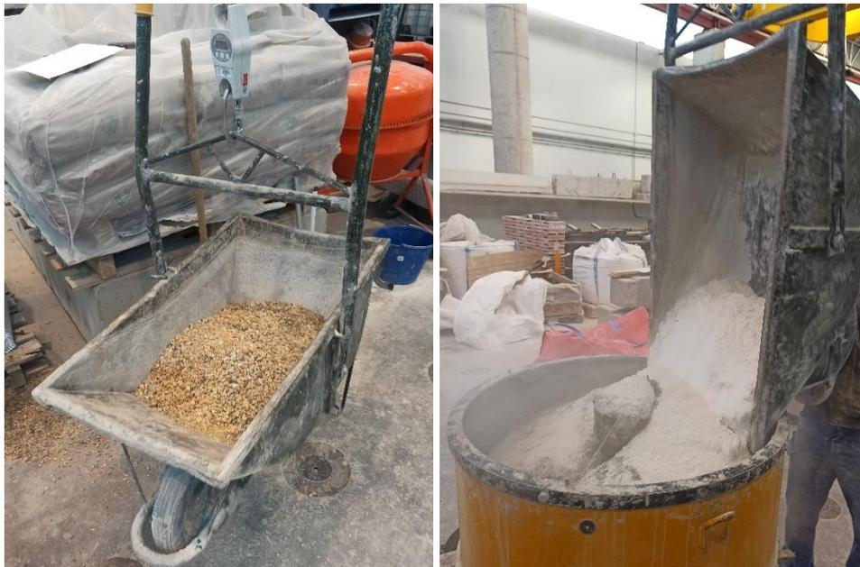
**Figure 3.1-6. Weighing of solid materials and pouring into the concrete mixer.**
