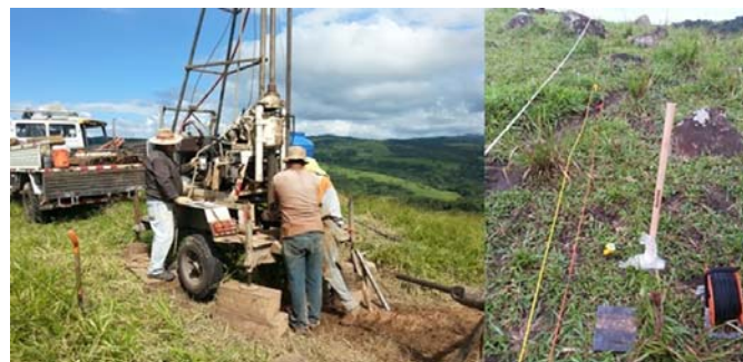
Figure 2. Equipment and tests carried out: SPT and seismic refraction tests.
