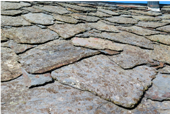
(a) Slates (Ardósia/Lousa) roof at Pinheiro Novo
