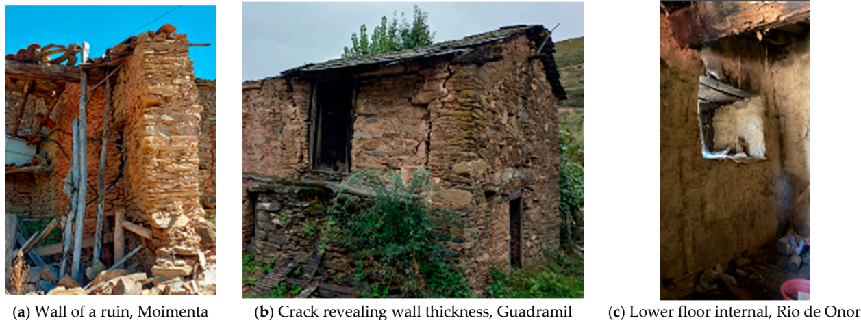
Figure 12. Thick masonry walls in MNP.
