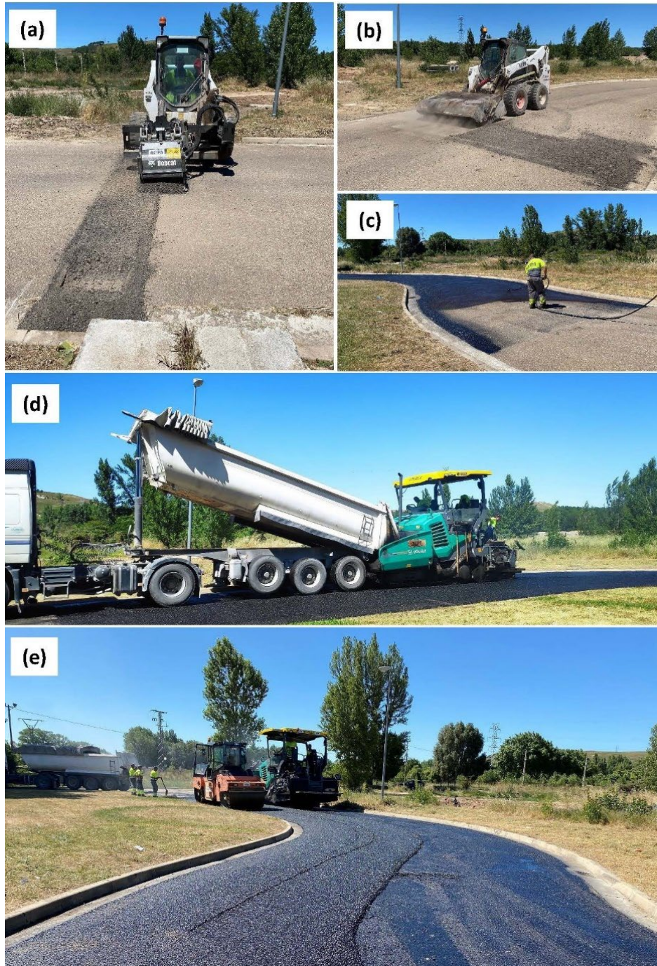
Figure 3. Construction of the pilot road section.
