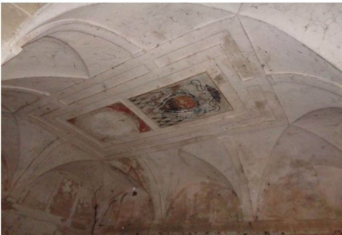
Fig. 3: Partitioned vaults over the main staircase. (Source: Imanol Ruiz de Vergara Ruiz de Azúa)
