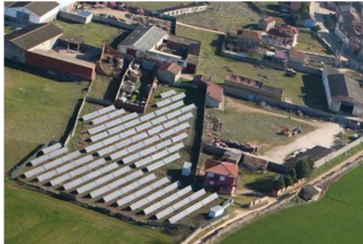
Figure 1. Aerial taken photograph of the facilities. Source [19].
