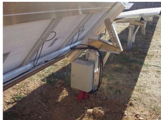
Figure 3. PV panels structures with hand-driven hor. axis regulation. Source [19].
