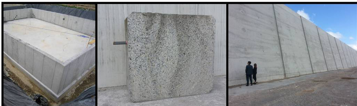
Fig. 1. Kubik building foundation and basement walls (left); a concrete block from the Punta Lucero dock (center) and the Punta Sollana dock wall (right), both at Bilbao Harbor (Spain).
