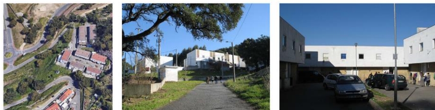
Fig. 5. Case study district. Aerial and general views of the neighbourhood.
