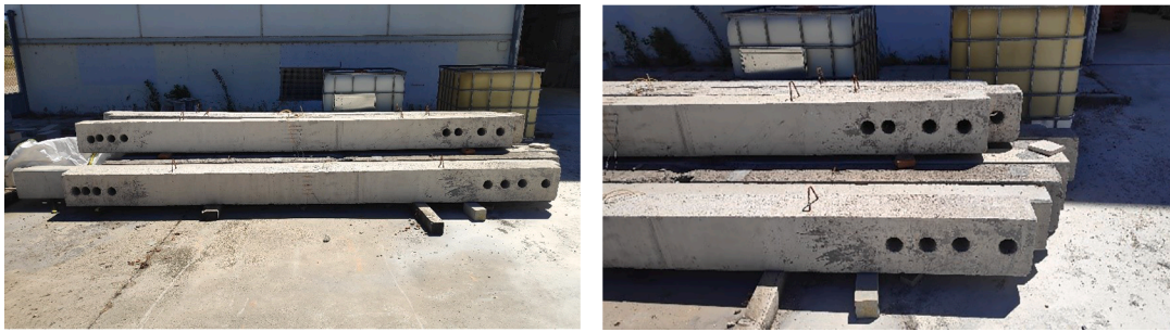
Fig. 3. Location of core drilling in the full beams (left) and detail of the ends of the beams (right).
