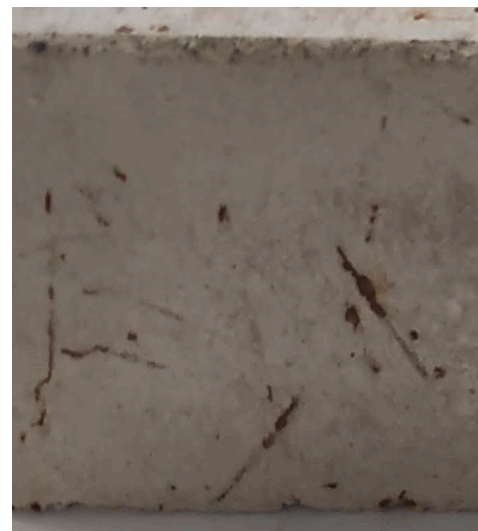
Fig. 17. Detail of the corrosion of external metallic fibers after the SO 2 -attack test on a mix SC/II-M specimen.
