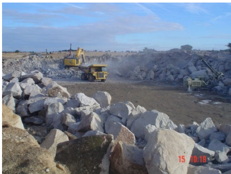
Figure 2. Granitic rock excavation associated to rockfill
