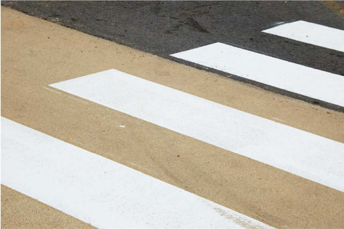
Fig. 17 – Crosswalk. Intersection between pavements.
