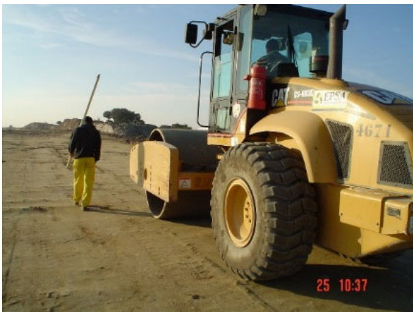
Figure 4. Topographic settlement control after roller pass
