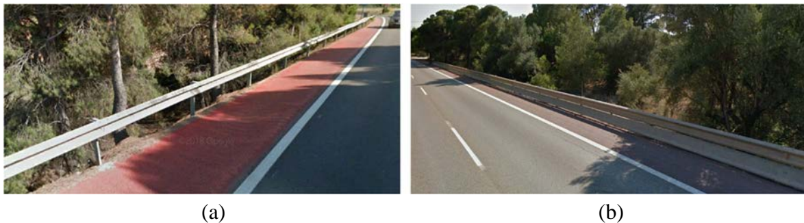
Fig. 5 - Lateral safety barriers observed in the study segment. (a) simple safety barrier; (b) double safety barrier.
