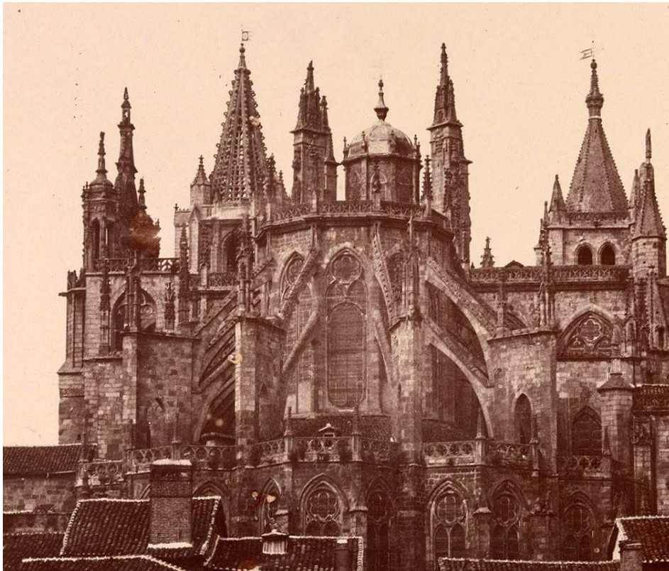
Fig. 10. Charles Clifford, Photograph of an exterior view of the rear of the Cathedral of Santa Maria de Regla in the city of León, https://www.rct.uk/collection/2700054/photographic-souvenir-of-spain-vol-i-view-of-the-cathedral-leon (consultado el 20 de abril de 2022).
