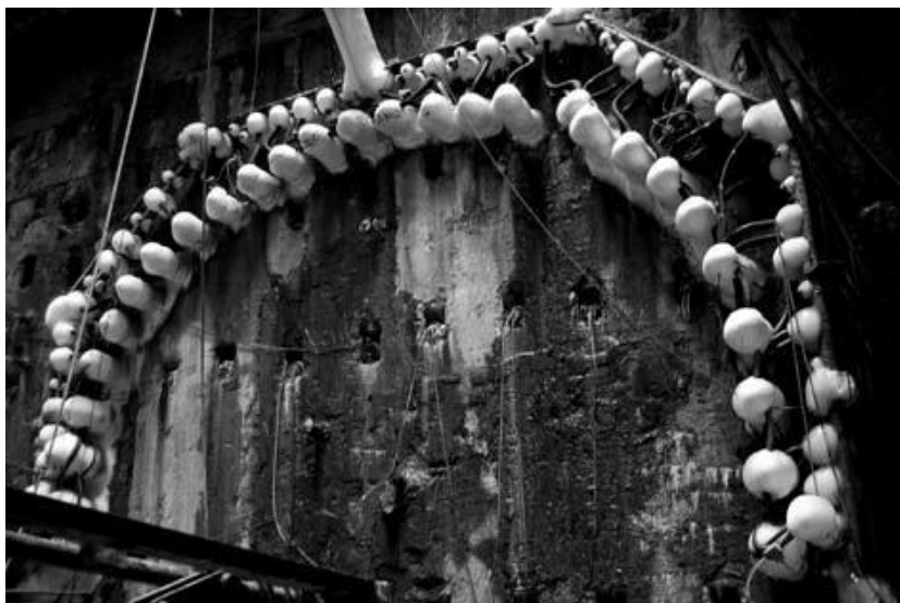
Figure 9.1: Overview of freeze pipe arrangement (Colombo, 2010)
