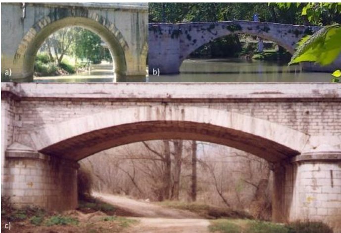
Figure 3. Three examples in the Carrion river basin (Spain). Upper left (a) Husillos Bridge (endings of 15 th century), a round arch; Upper right (b) Villoldo Bridge (endings of 18 th century), a semi-shallow arch; below (c) San Isidro Bridge in Dueñas (early 20 th century), a shallow arch.
