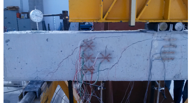
Fig. 4. Left shear span of the IP beam.
