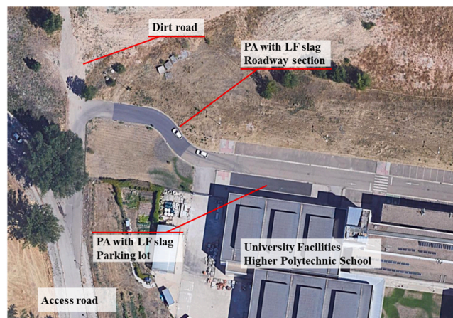
Fig. 3. Aerial view of the pilot project.
