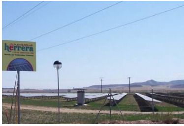
Figure 2: System 1 facility located at Herrera de Valdecañas (Palencia, Spain)
