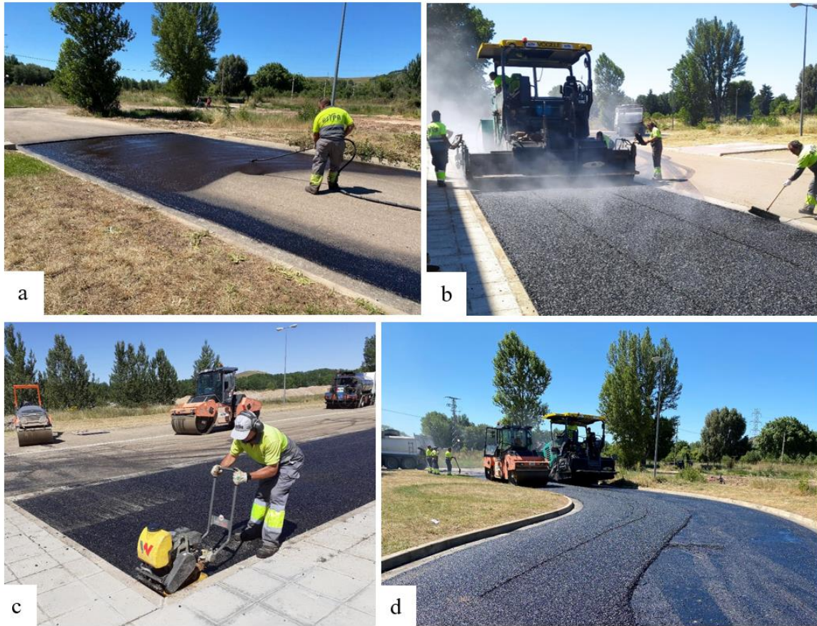
254 Figure 3. (a) Surface preparation. (b) Paving the parking area. (c) Manual border 255 compaction. (d) Laying and compacting on the roadway section.
